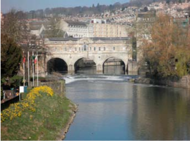
Pulteney weir and radial gate
