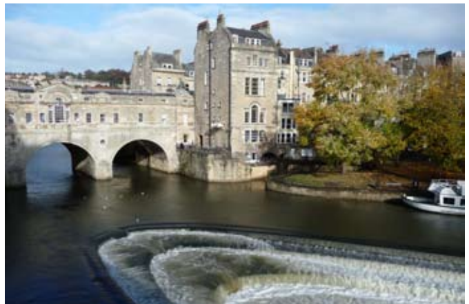
Pulteney Bridge and Weir, Bath
