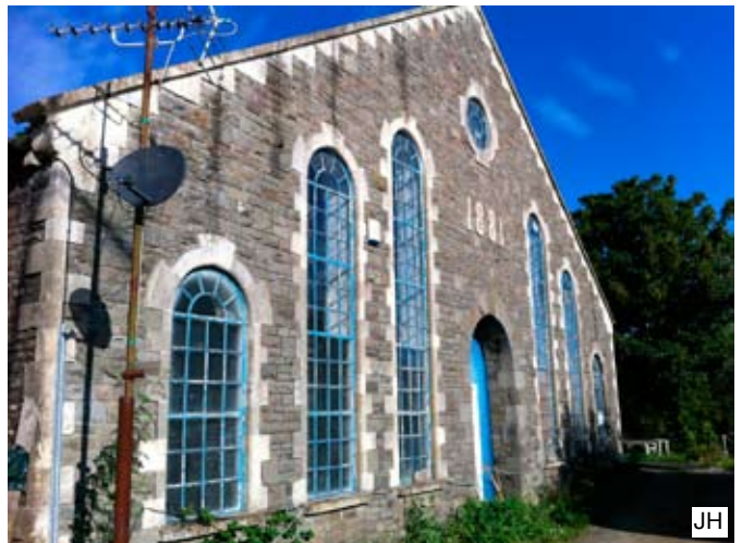
Old Polysulphin Factory Building, Keynsham
